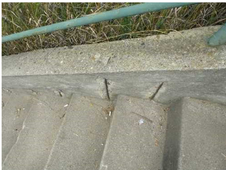
DTTO - drobné poruchy.
